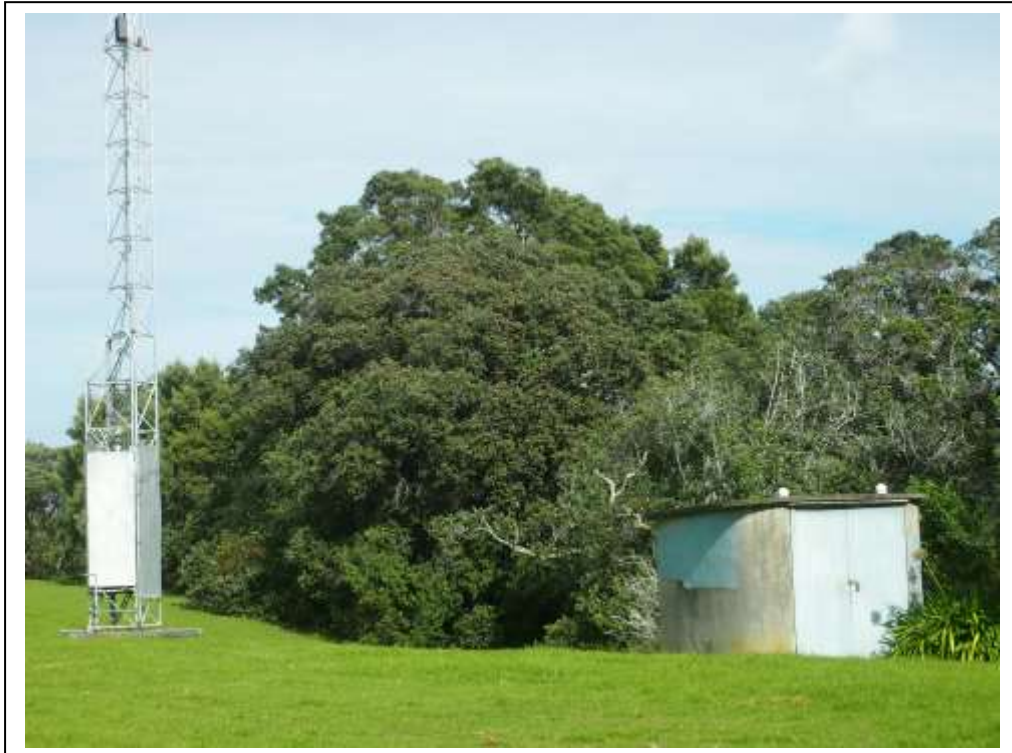
Figure 6: Concrete outbuilding and west radio tower, Musick Memorial Radio Station, Auckland, 5 May 2015. Karen Astwood, IPENZ.
